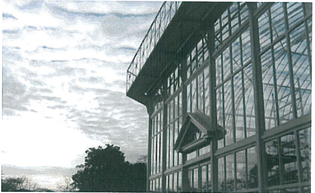
The Great Palmhouse at the National Botanic Gardens: 28,000 metres of a very specialised form of MS polymer sealant were used for the glazing, to metal and teak, coated with both polyurethane and acrylic paints.
